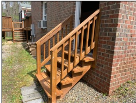
No Landing Observed
