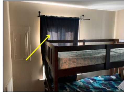
The Upper Sash of this Window in the Downstairs Rear Right Bedroom has Condensation Between the Panes
