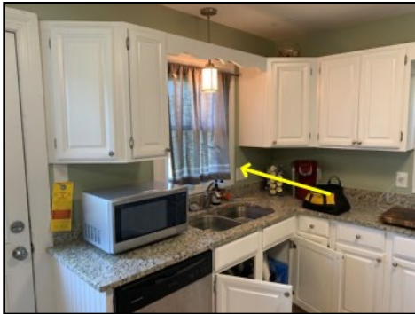
The Lower Sash of this Window in the Kitchen has Condensation Between the Panes
