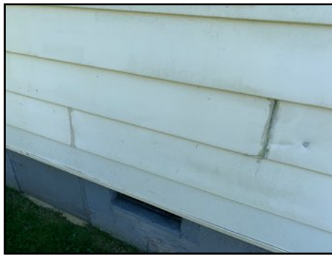
Caulking/Inadequate Sidelap
