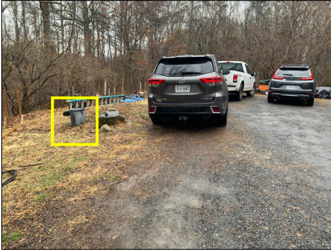
Below Grade Propane Tank Located Here
