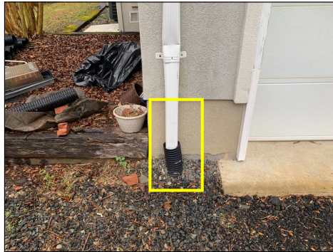
Downspout Terminating Below Grade (Representative Photo)
