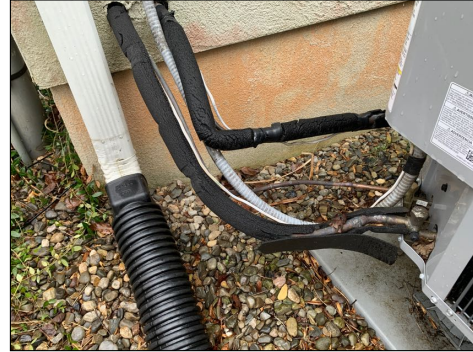
Condensate Drain Line too Close to Foundation Damaged/Missing Insulation at Refrigerant Lines
