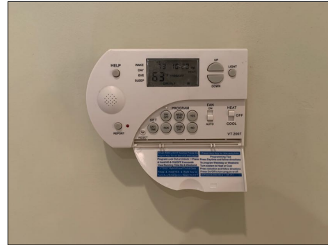
General Photo (Second Floor)
