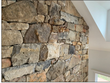
Efflorescence Observed
